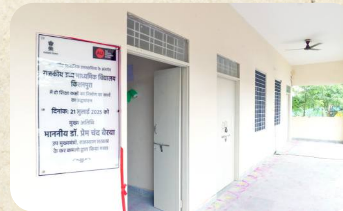
Classroom constructed at a government school in Dudu
