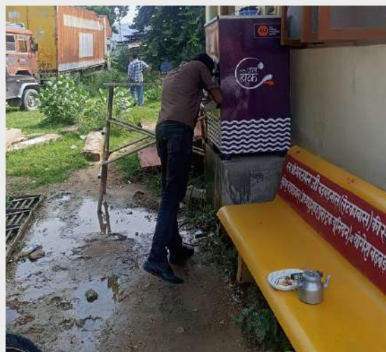
Image: Stagnat water at one of the water coolers
