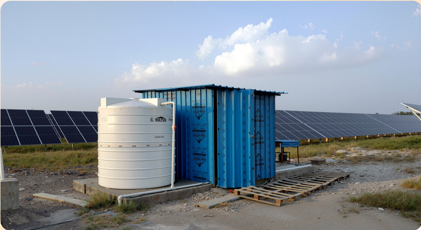
A bathroom for the plant staff Site: UV Solar, Jaipur District
