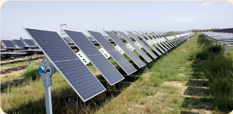
Solar Panels follow the sun's trajectory Site: Supyar Kanwar, Jaipur District
