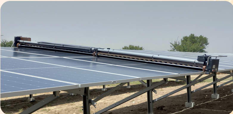
Automatic cleaner cleans panels without using water Site: Anjani Renew Agro, Jaipur District
